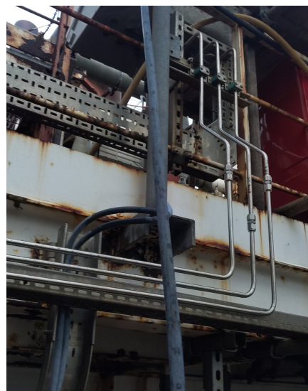
Examples of fabricated, strength tested, and installed SBT assemblies
