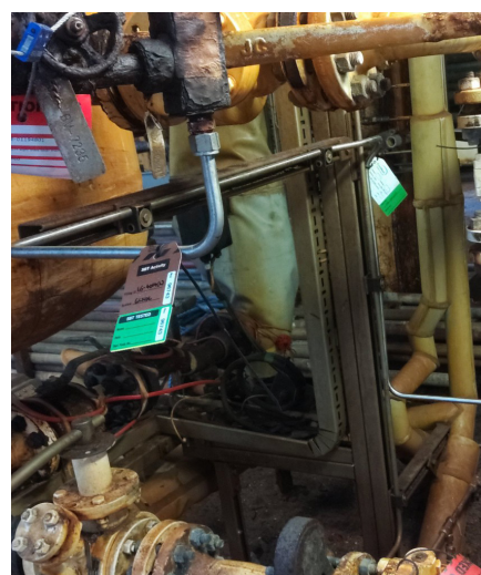
Examples of fabricated, strength tested, and installed SBT assemblies
