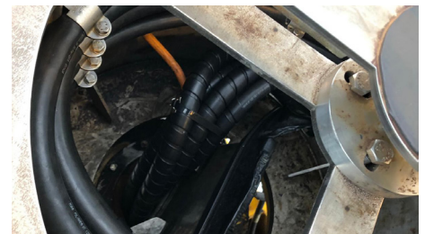
Technician Terminating Cables
